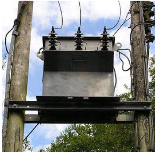
Gambar 2.2 Transformator Distribusi 3 fasa
