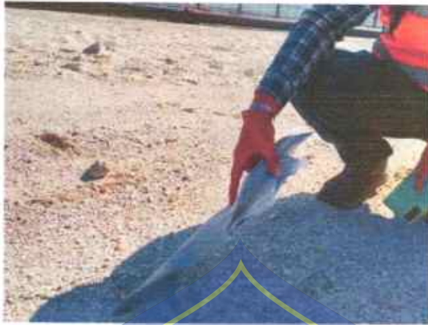
PVD (Prefabricated Vertical Drain)
