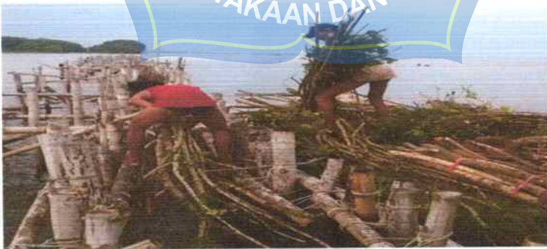
Gambar 11. Proses pengisian ranting di struktur HE (Sumber Gambar: Ecoshape Consortium, 2016 )
