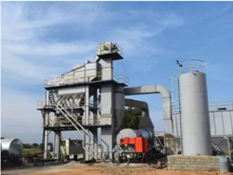
Gambar 12.7. Asphalt Mixing Plant. (Erwin 2022).
