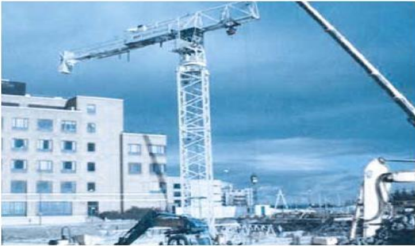
Gambar 6. 1 Peralatan Bangunan (Sumber: www.pogo.org.uk )
