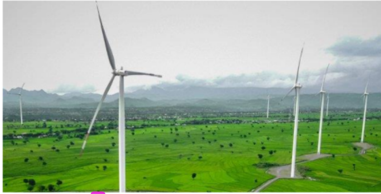
Fig.3. Wind Power Plant in Jenepono, South Sulawesi.
