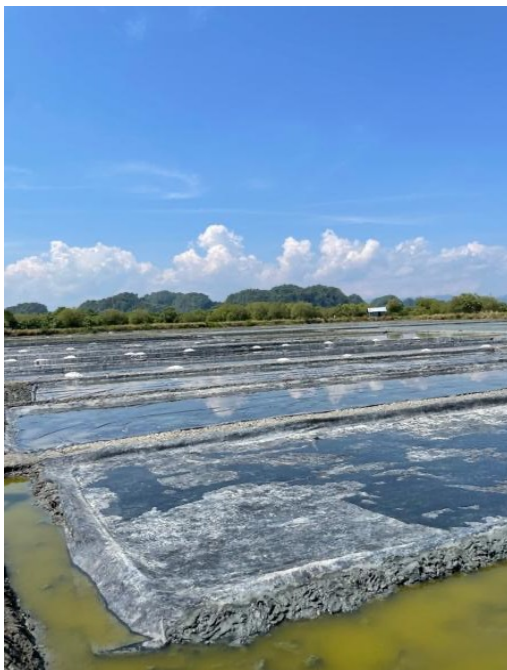
Figure 2. Use of geomembrane technology in salt ponds in Bulu Cindea Village, Bungoro Sub-district, Pangkep Regency
