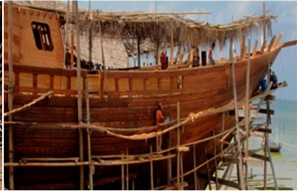
(b) The Finishing Process of Pinisi
