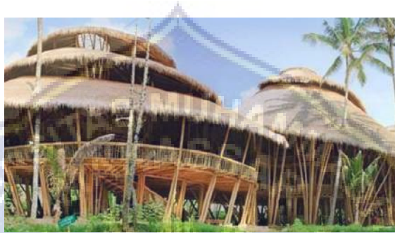
Gambar 2.8 Fasad Bangunan Green School Bali (sumber: https://www.greenschool.org/ .2022)
