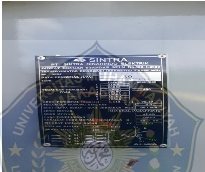
GAMBAR 4. 6 Name plat Trafo Distribusi BMGX BT50-087 (ulp tanete up3 bulukumba)
