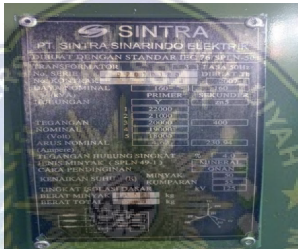
Gambar 4.4 Nameplate transformator distribusi sintra
