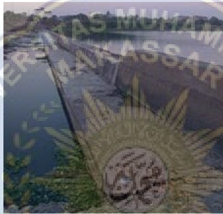
Gambar. Model bangunan groundsill
