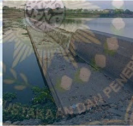
Gambar 3. Model bangunan groundsill
