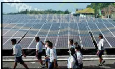
Gambar 9. Panel Surya ( https://alamendah.org/2energi-surya-matahari-di-indonesia )
