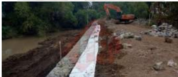
Gambar 2.11 Penerapan Dinding Penahan Geotextile Non Woven
