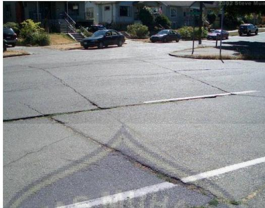
Gambar 5. *Joint Reflection Cracking*
