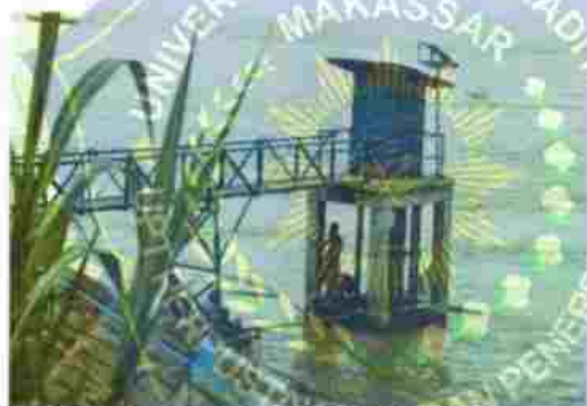
Gambar 2.6 (Gambar Pos Duga Air)
