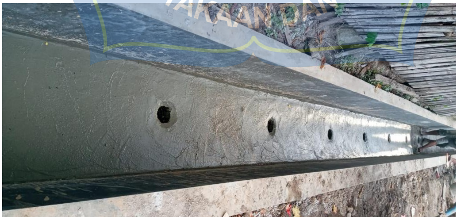
Gambar 4 Drainase Biopori
