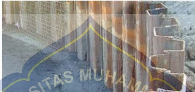
Gambar 6 Steel Sheet Pile Seawall (Sumber: Indriyani R., 2019)
