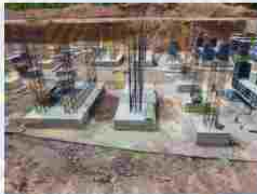
Gambar 19. Gambar Pondasi Foot Plat Sumber: https://www.archify.com/id
