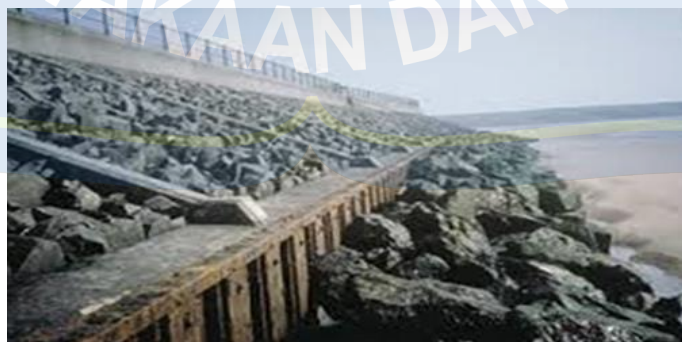
Gambar 7 Concrete Block and Rock Walls (Sumber: Indriyani R., 2019)
