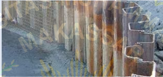
Gambar 6 Steel Sheet Pile Seawall (Sumber: Indriyani R., 2019)
