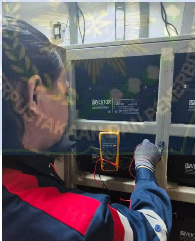
Pengukuran Floating Battery (Tanpa Beban)
