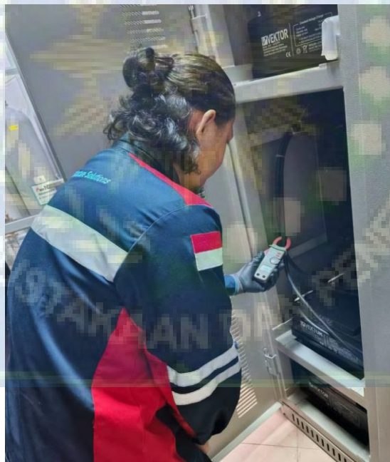
Pengukuran Arus Battery
