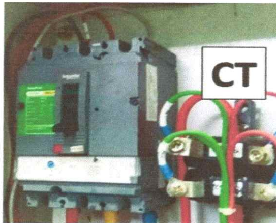
Gambar 2.13 Current Transformar
