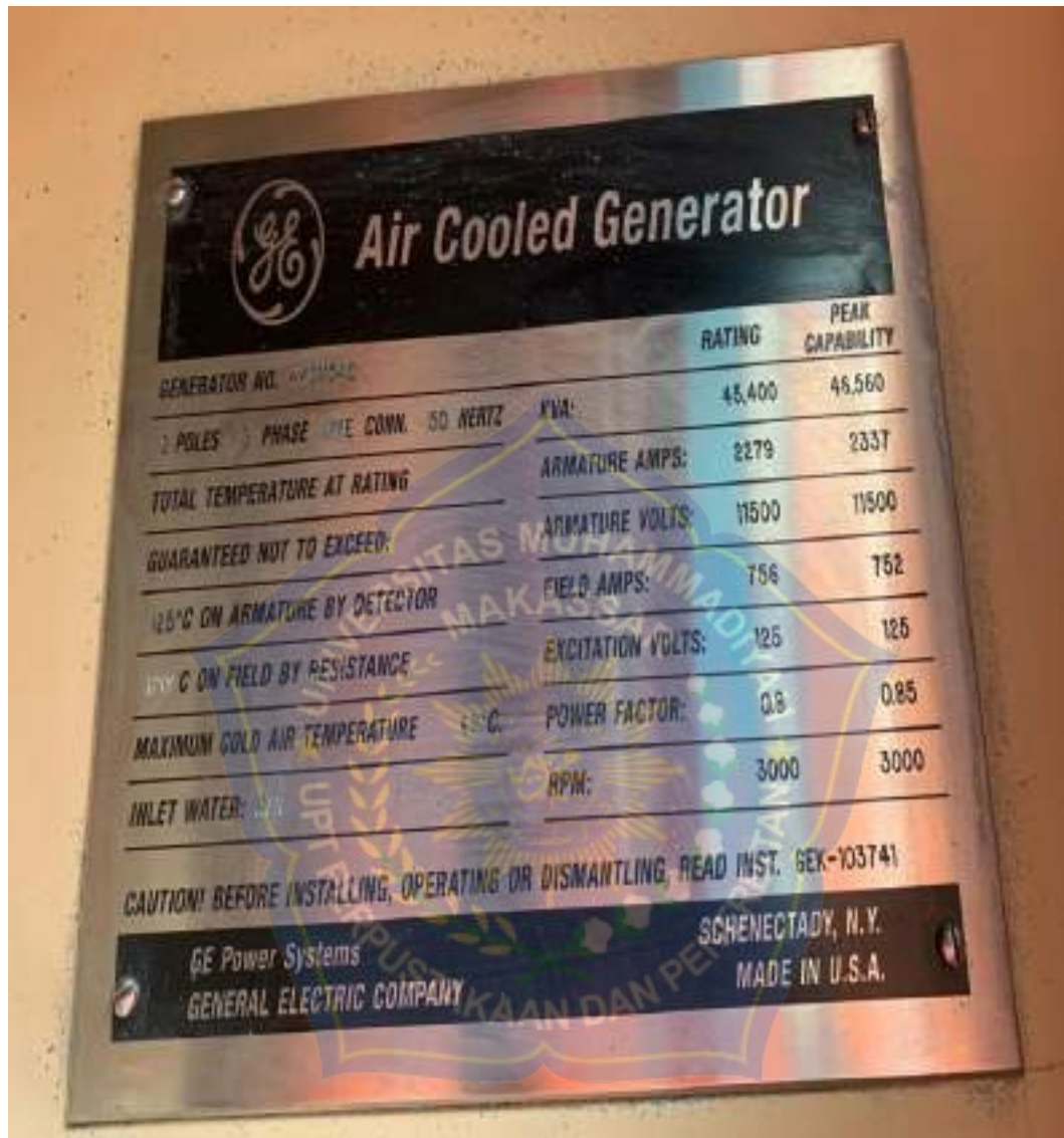
Lampiran B.1. Data Generator #GE1 PLTG Tello (PLN, 2025)
