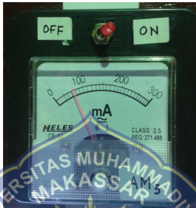
Gambar L.23. Arus netral lampu TL 10 Watt
