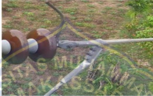
**Gambar 2.7** jumper *joint*
