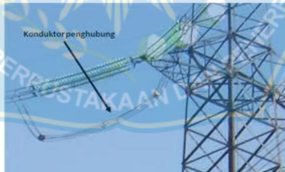
**Gambar 2.8** jumper *conductor*
