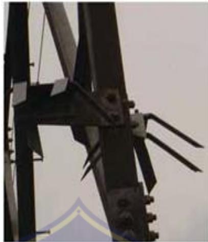
**Gambar 2.18** Anti *Climbing Device* (ACD)
