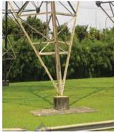
**Gambar 2.14** Pondasi tower (*lattice*) SUTET 500 kV Gresik - Krian
