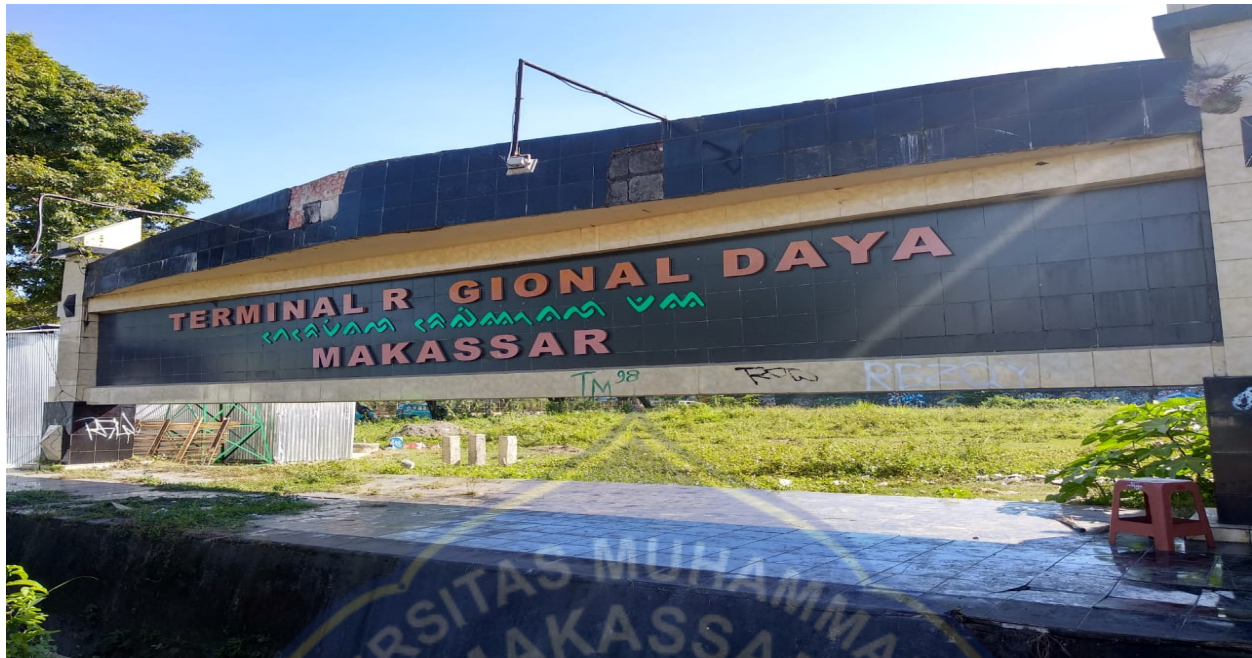
TERMINAL REGIONAL DAYA
