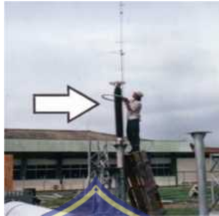
Gambar 2.20. Lightning Arrester (LA) .
