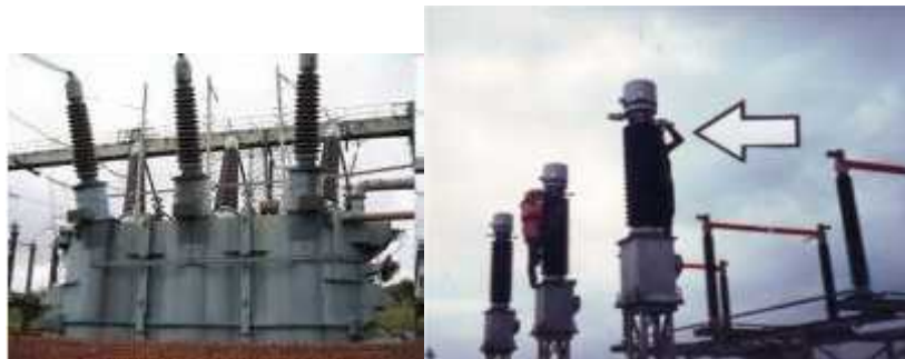
Gambar 2.17. Trafo Arus { Current Transformer (CT) }.
