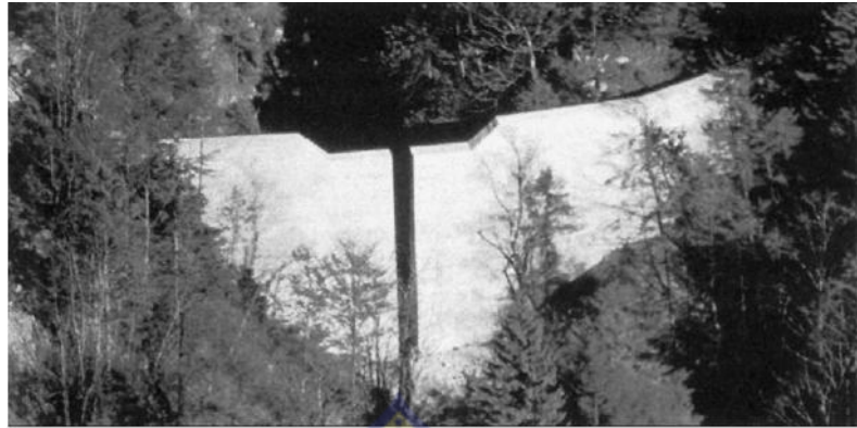
Gambar 8. Check Dam Tipe Slit.
